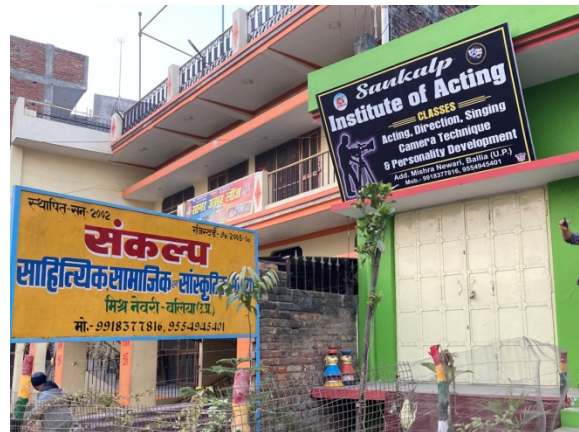
Figure 49 The 'Sankalp' building
